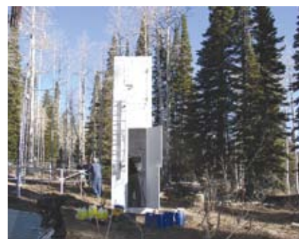
Summer maintenance on a SNOTEL site.
