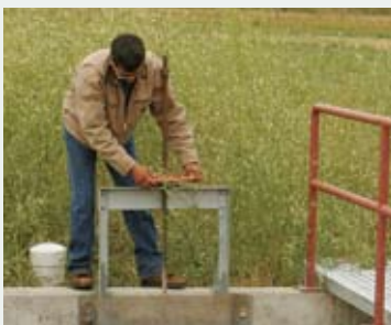
Gates allow producers to control irrigation water to their fields.
