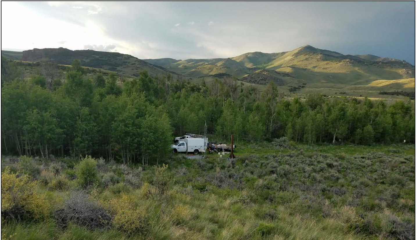
O'Neil Creek SNOTEL site installation in the Salmon Falls basin, June 6, 2018.
