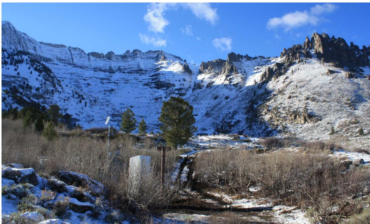
Photo 1: Hole in Mountain SNOTEL in its new location. The site is tucked behind a small ridge about 450ft south of the original location. This new location will keep future avalanches from impacting the site. Photo taken October 2016.
