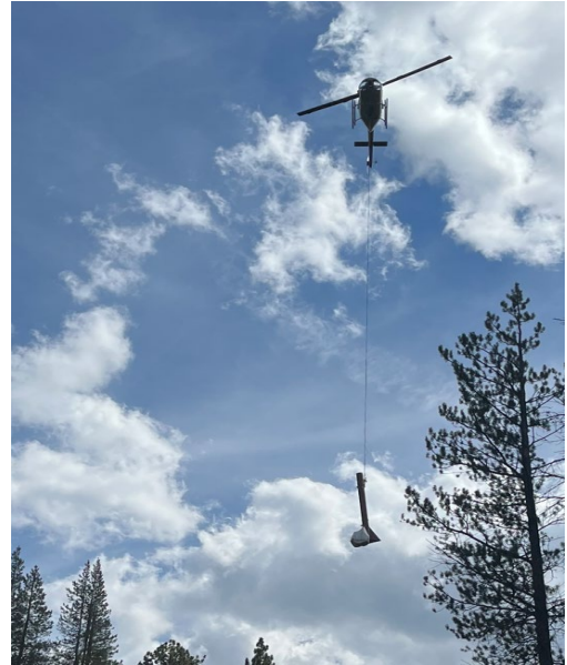
Figure 2: Flying a taller precipitation gage into Poison Flat SNOTEL.
