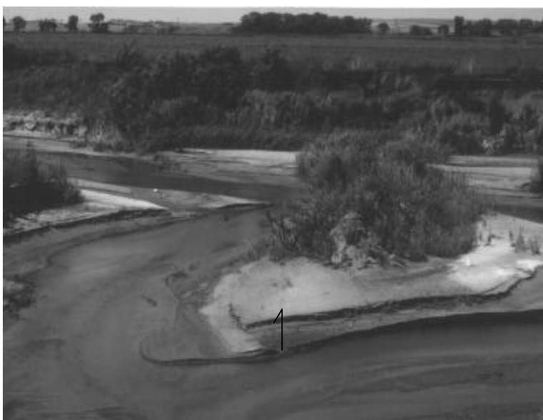
Figure 1. Sugar Creek shown 3 miles north of Gracemont illustrates extensive channel widening and readjustment. Remnants of jacks on the left side of island mark the edge of stream at some time in the past.
