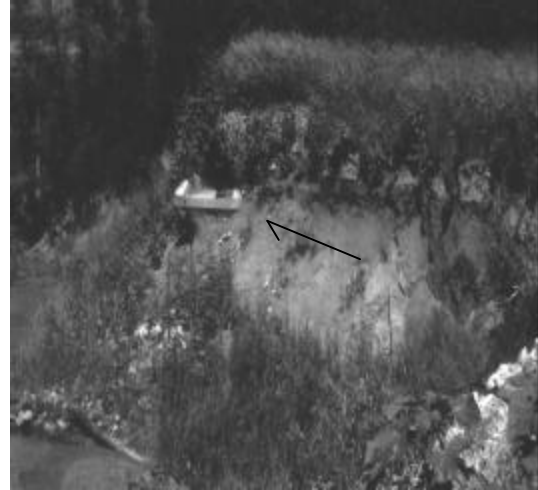
Figure 8. Note location of concrete pad for road culvert relative to current stream location and lack of vegetation in the midbank region.
